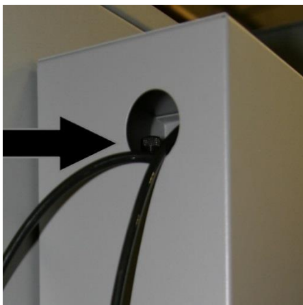
Figure 8: Water Lines Threaded
